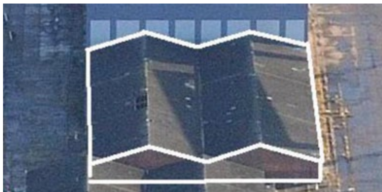
Building 14 & 13 Fabrication Halls
