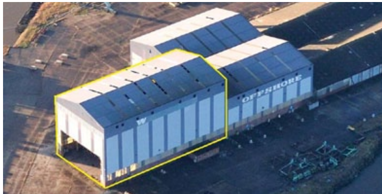
Building 19 Large Fabrication Hall 58m x 30m 27.8m Eaves
